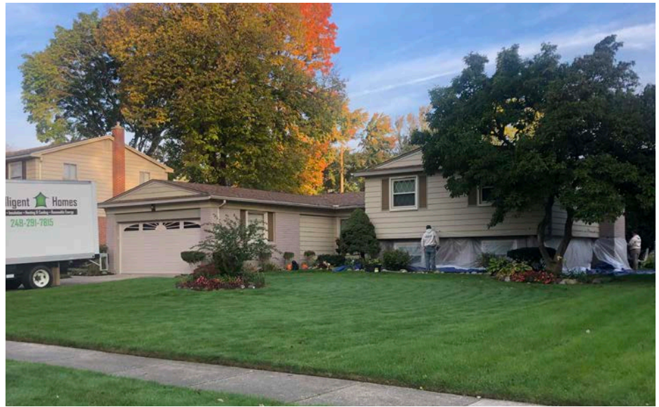
With minimal insulation and no air sealing, Margaret Rankin's split-level home had some serious comfort issues.
