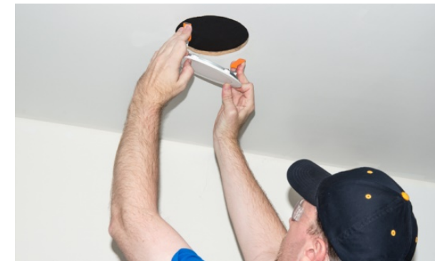
Install fixture fitting in ceiling using (2) integral mounting springs
