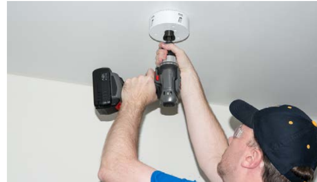
Cut Hole In Ceiling
