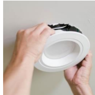
Squeeze and Insert Torsion Springs/Friction Blades
