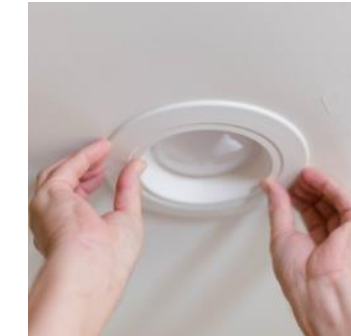
Guide LED Module into Recessed Housing
