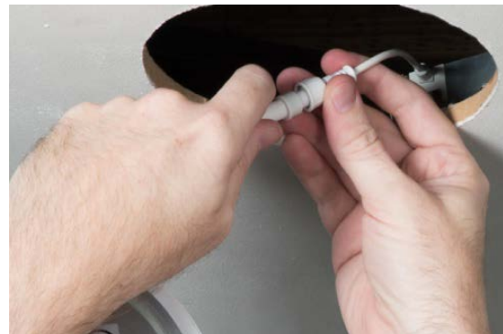
Connect in-line plenum rated connector
