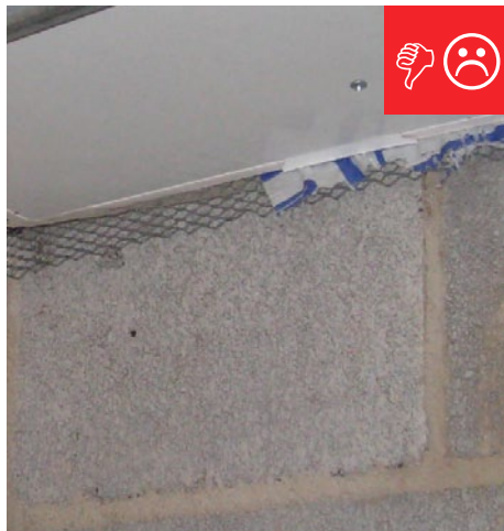
C. The water-resistant barrier, weep screed, and stucco lathe are not properly layered.
