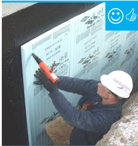
Below-grade concrete has been properly sealed against moisture and is now having insulation installed.
