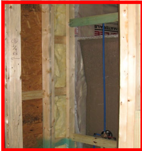
A. No backing installed behind shower enclosure.
