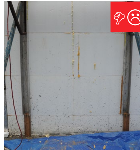
D. The insulated concrete forms at the foundation do not have a damp-proof coating.
