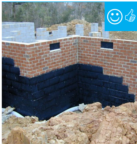
The below-grade concrete walls have damp-proof coating.
