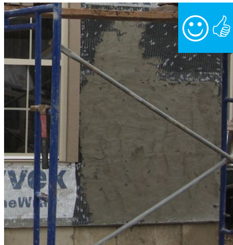
The water-resistant barrier, weep screed, and stucco lathe are properly layered and will create a complete drainage system.
