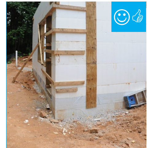
The insulated concrete forms that are below grade have a damp-proof coating to prevent moisture seeping into the foundation.
