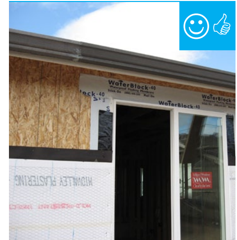
There is a water-resistant barrier installed underneath the stucco and lathe.
