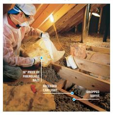
Cut a 16 inch long piece from a batt of unfaced fiberglass insulation and fold it into the bottom of a 13-gallon plastic garbage bag.
