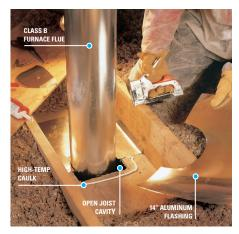
Cut aluminum flashing to fit around the flue. For round flues, cut half circles out of two pieces so they overlap about 3 inches in the middle. Press the flashing metal into a bead of high-temperature caulk and staple or nail it into place. If there's no wood, staple or nail it directly to the drywall, but be sure not to staple or nail through the drywall.
