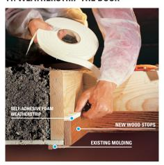
Weatherstrip the attic access hatch or door. Cut 1x3 boards to fit the perimeter of the opening and nail them on with 6d finish nails. Apply self-adhesive foam weatherstrip tape to the top edge of the stop.
