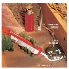
Fill wiring and plumbing holes with expanding foam.
