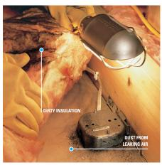
Check for gaps in your attic that facilitate air movement by checking for dirty insulation. Seal the gaps with caulk or expanding foam. When complete and dry, push the insulation back into place.
